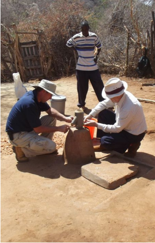
Colin Martin and Adrian Moore fitting the Canzee pump at Kandongu Well
